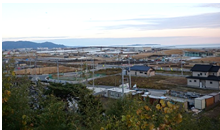
Reconstruction project site of Kadowaki and Minamihama area, Ishinomaki City's largest disaster area.
